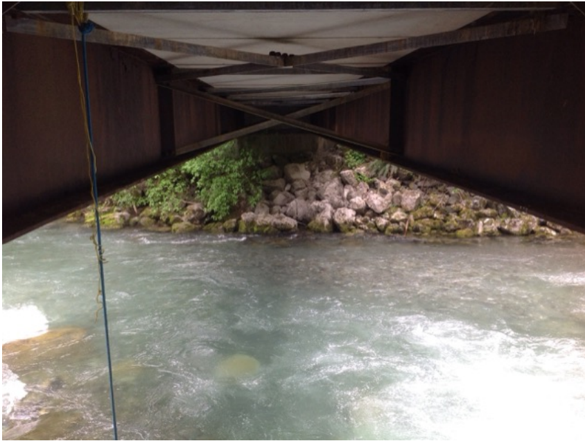
Right Bank Abutment when facing downstream
