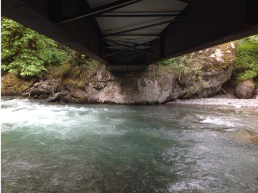
Left Bank Abutment when facing downstream
