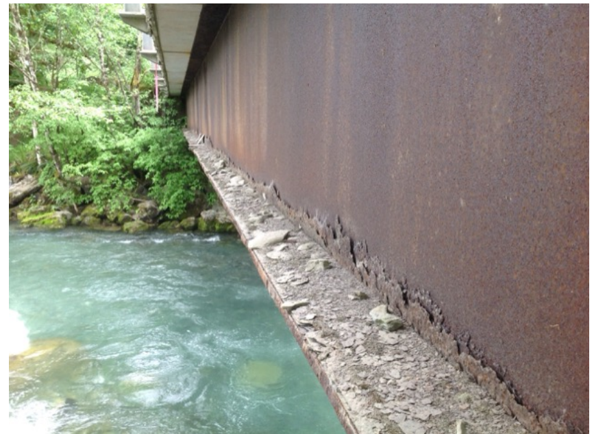
delaminating steel
