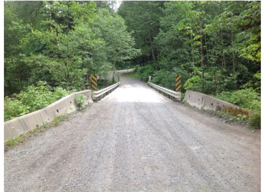
Approach from Left Bank when facing downstream
